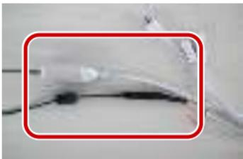
3. Protect other cables using insulating tapes.
